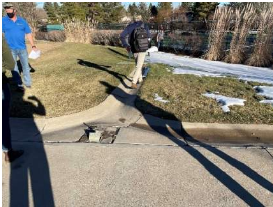
SWALE TO TENNIS COURT WALL
