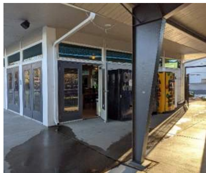
Drainage at North East Corner
