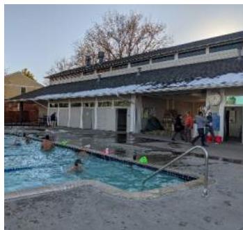
East Façade at pool
