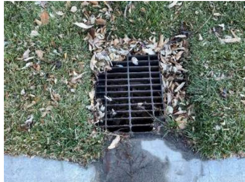
CATCH BASIN ADJACENT TO POOL DECK
