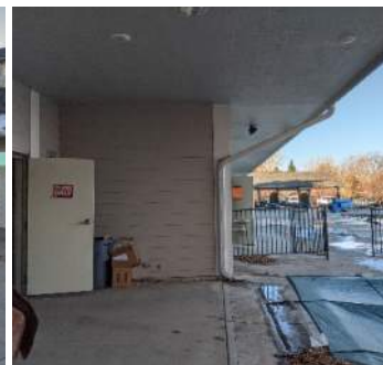
South East Corner Overhang
