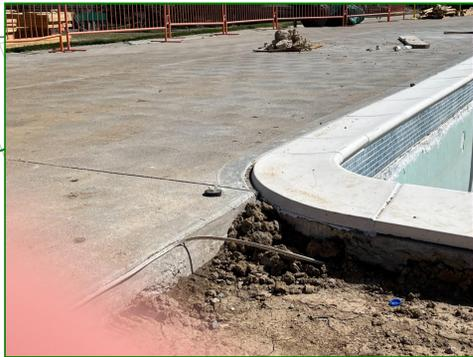
When the new coping was installed at the lap pool, the waterline side of the coping was placed level in order to keep the waterline tile level. As a result, some coping stones are raised above the pool deck. The worst elevation difference is 1" at the SE corner.
